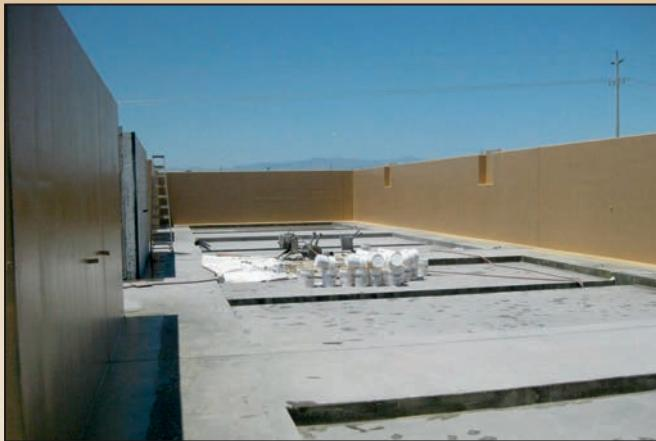
**SewerGard® 210T - Trowelable** is an aggregate-filled epoxy. Its non-sagging consistency makes it the material of choice for vertical and overhead surfaces or where access is limited. Standard application thickness is  $\frac{1}{8}$ ".
