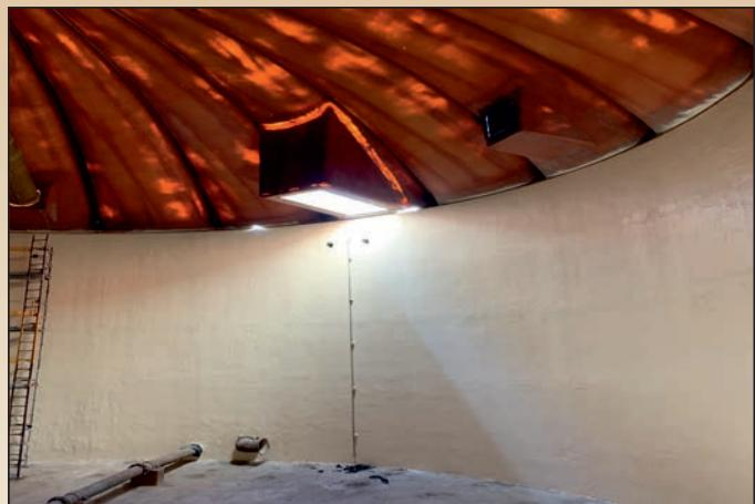
**SewerGard® 210X - High-Strength** is a high-strength lining that enables high-build capabilities wherever extreme corrosion conditions exist. Applied by plural-component or conventional airless spray equipment up to 65 mils per coat, or greater depending upon surface conditions, application technique, application equipment and exposure.
