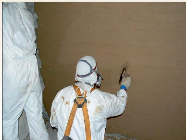
**SewerGard® 210S - Sprayable** is fiber-reinforced for a high degree of durability. 210S allows quick installation in a single 60 mil coat when applied by standard airless equipment. It is ideal for large-scale applications.
