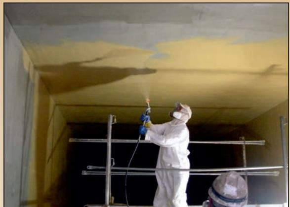
**SewerGard® 210RS - Rotary Spray** is specifically designed to line the interior of an 8' deep manhole from street level in less than 20 minutes. 210RS is applied up to 125 mils using typical rotary application equipment.
